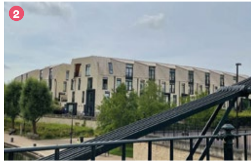
Looking south-east from Victoria Bridge
