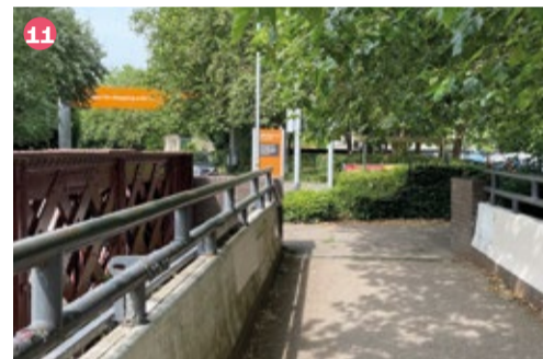
View west on footbridge
